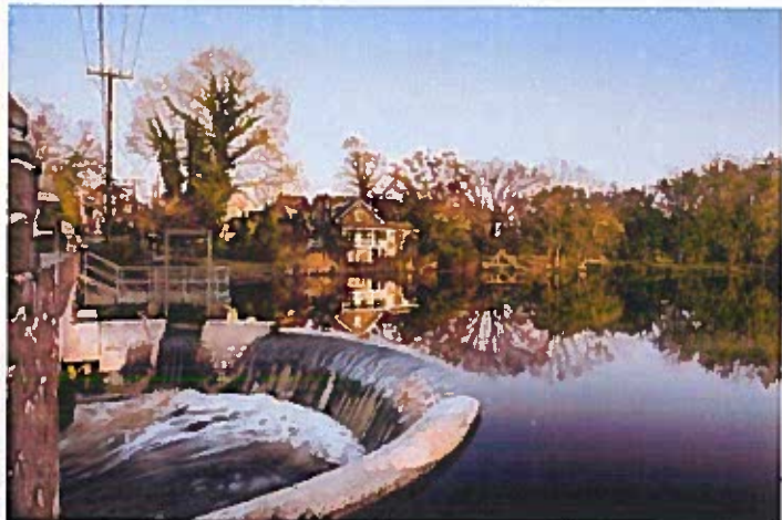
Figure 2 Race Street Spillway in Vincentown
